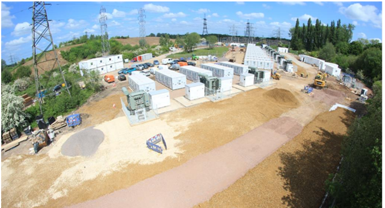
Plate 3.10: Example of the Construction of BESS Compound
